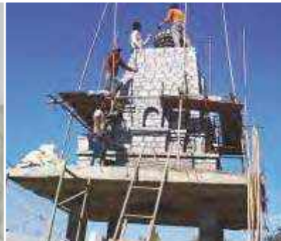
Const of dome by Flyocrete A.A.C. Blocks
