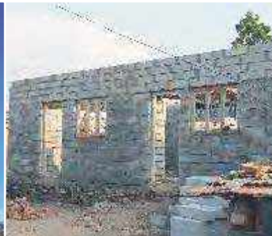
Villager's Home constructed by using Flyocrete Blocks under Govt. Scheme
