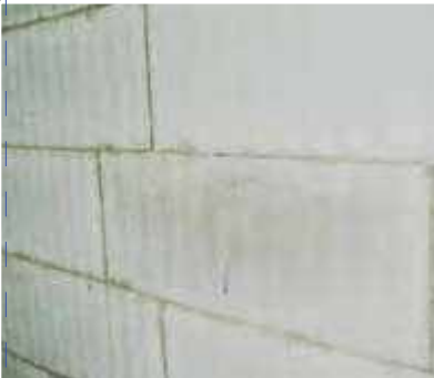
Actual Photograph of Flyocrete Blocks Joints filled with Flyobond Dry Mortar
